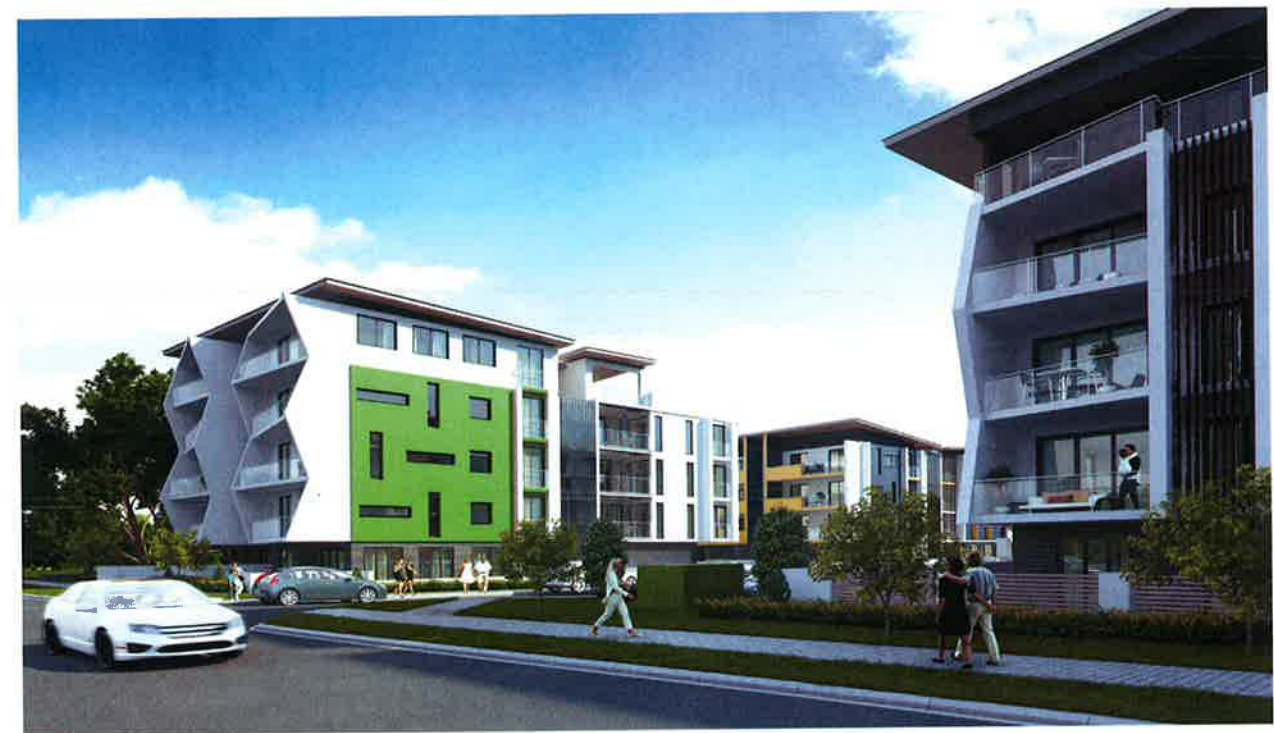
VIEW FROM RYNAN AVENUE - FACING TO SOUTH WITH BUILDING A TO RHS, BUILDING B TO LHS & BUILDING C IN CENTRE
